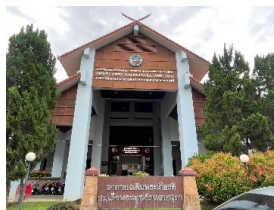
Princess Maha Chakri Sirindhorn Building
