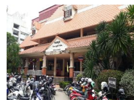
Wiphat Boonsri Wangsai Building
