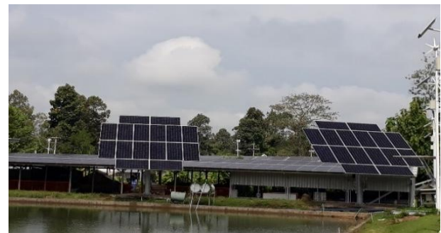
A solar tracking station with a capacity of 20 kW has been erected.
