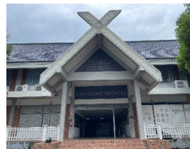
Thep Sat Sathit Building
