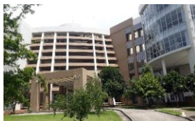
Architecture and Environmental Design Building (New)
