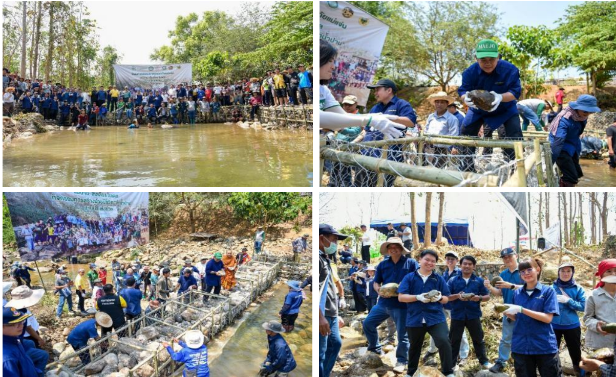
Water retardation weir construction project
