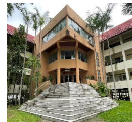
Architecture and Environmental Design Building
