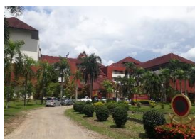
Engineering Laboratory and Classroom Building
