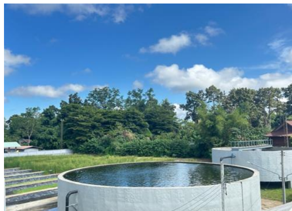
Primary and secondary wastewater treatment system : SBR
