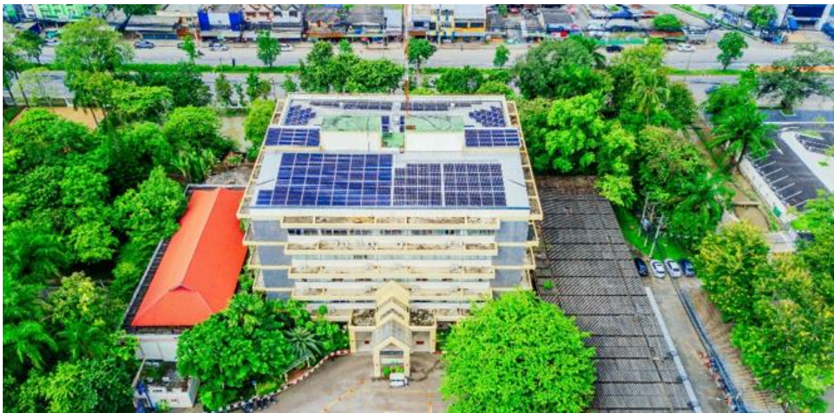
Solar rooftop with a 110-kW installed capacity
