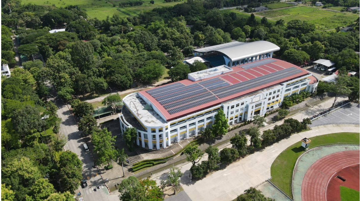
Installation of rooftop solar systems on buildings and student dormitories
