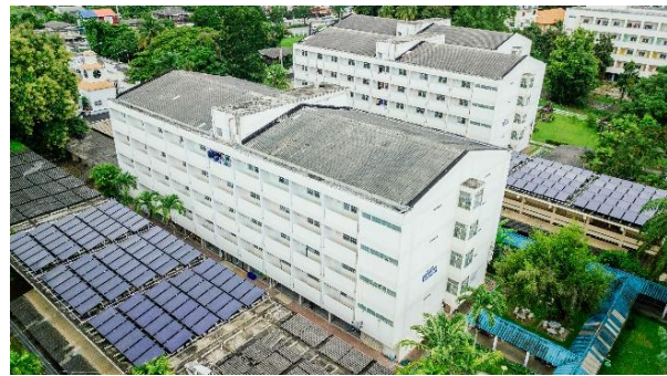
tanks atop the students' dorm and solar collectors with a 1331 m 2 installed capacity
