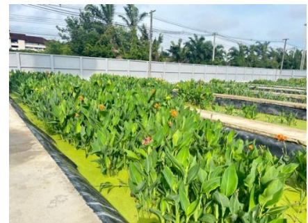
Wastewater treatment plants by constructed wetland
