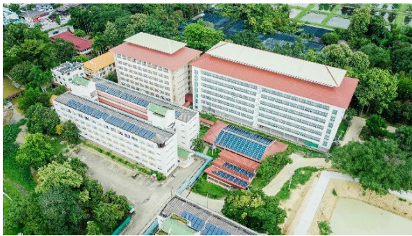
tanks atop the students' dorm and solar collectors with a 1331 m 2 installed capacity
