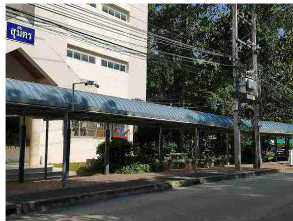
CCTV cameras around the university's dormitories areas
