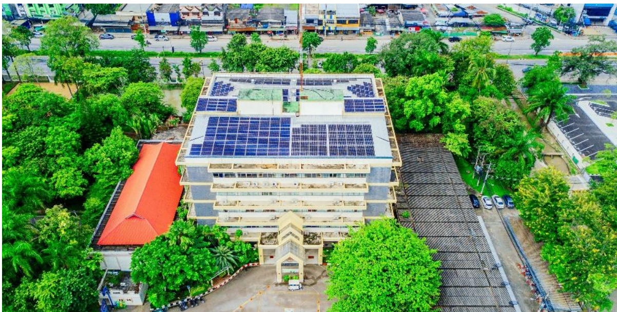
Solar rooftop with a 110-kW installed capacity
