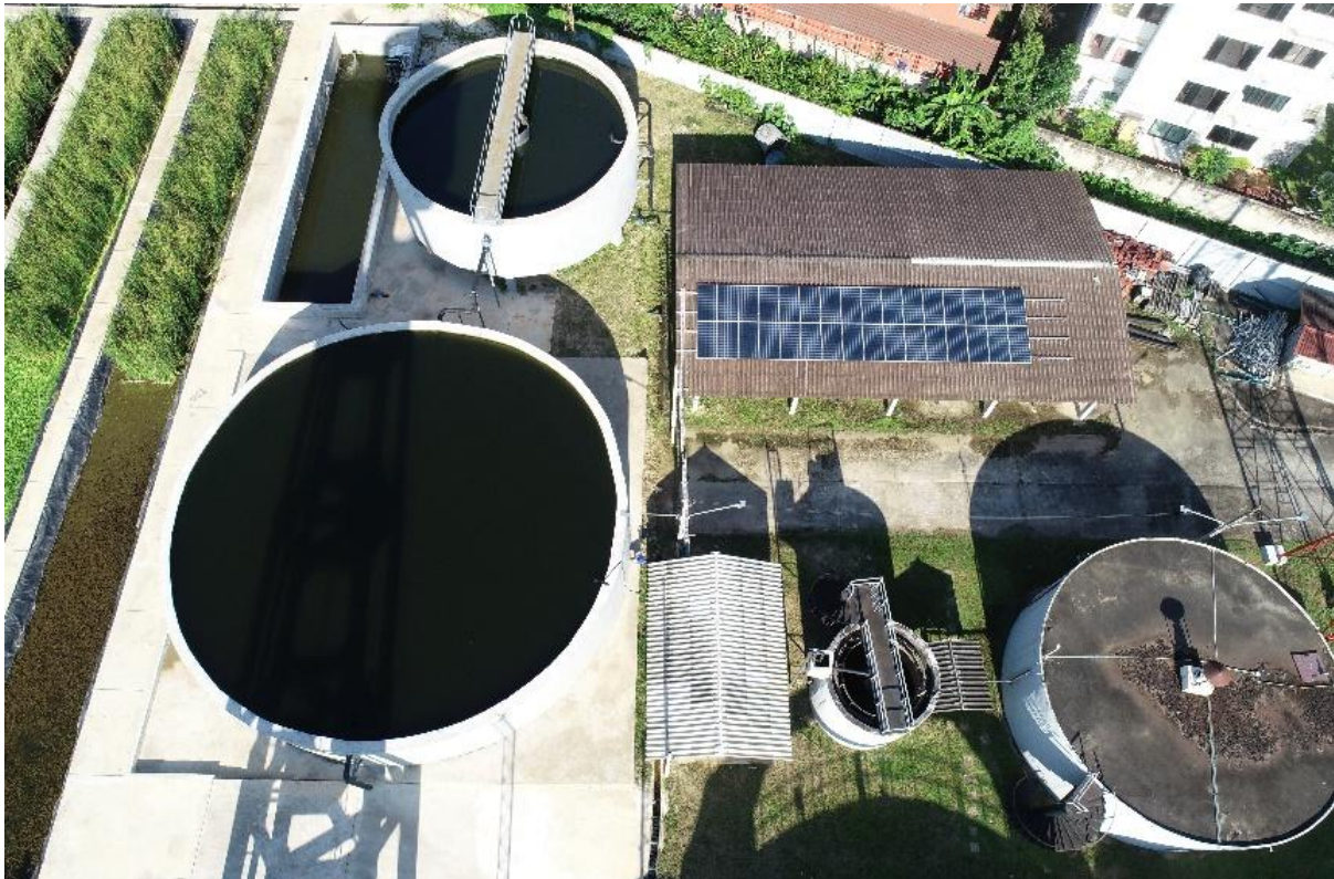
Solar panels with 10 -kW installed capacity on the roof Wastewater treatment
