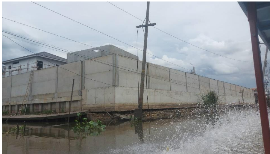
Figure 3 Physical separation between riverside and new communities by constructed high walls
