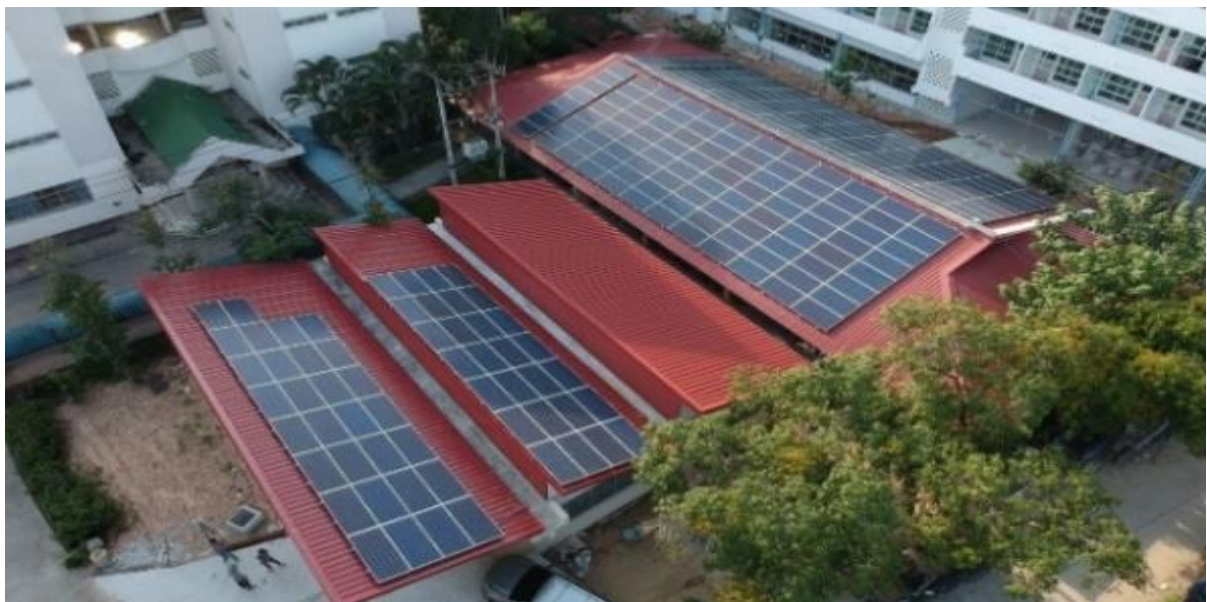
Solar rooftop with 80-kW installed capacity
