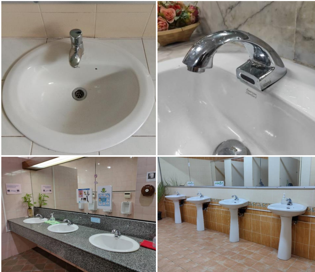
Low flow taps and automatic taps
