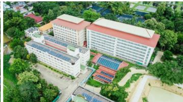
Tanks atop the students' dorm and solar collectors with a 1331 m2 installed capacity
