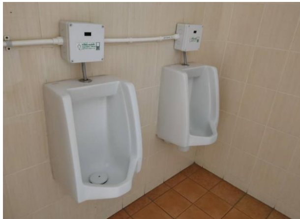
Waterless urinals and automatic urinals
