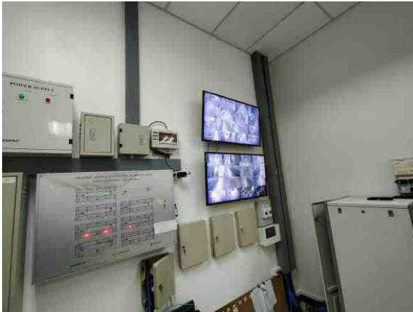
Graphic Annunciator informs the location of the incident in the building
