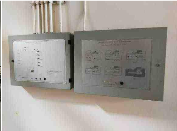
Graphic Annunciator informs the location of the incident in the building
