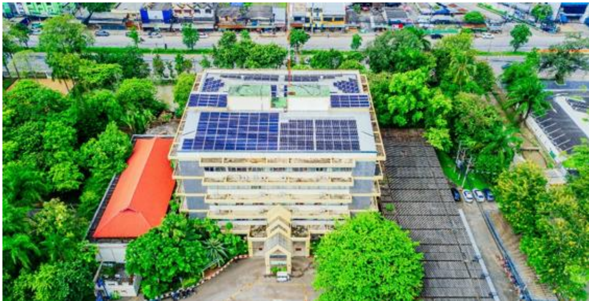
Solar rooftop with a 110-kW installed capacity
