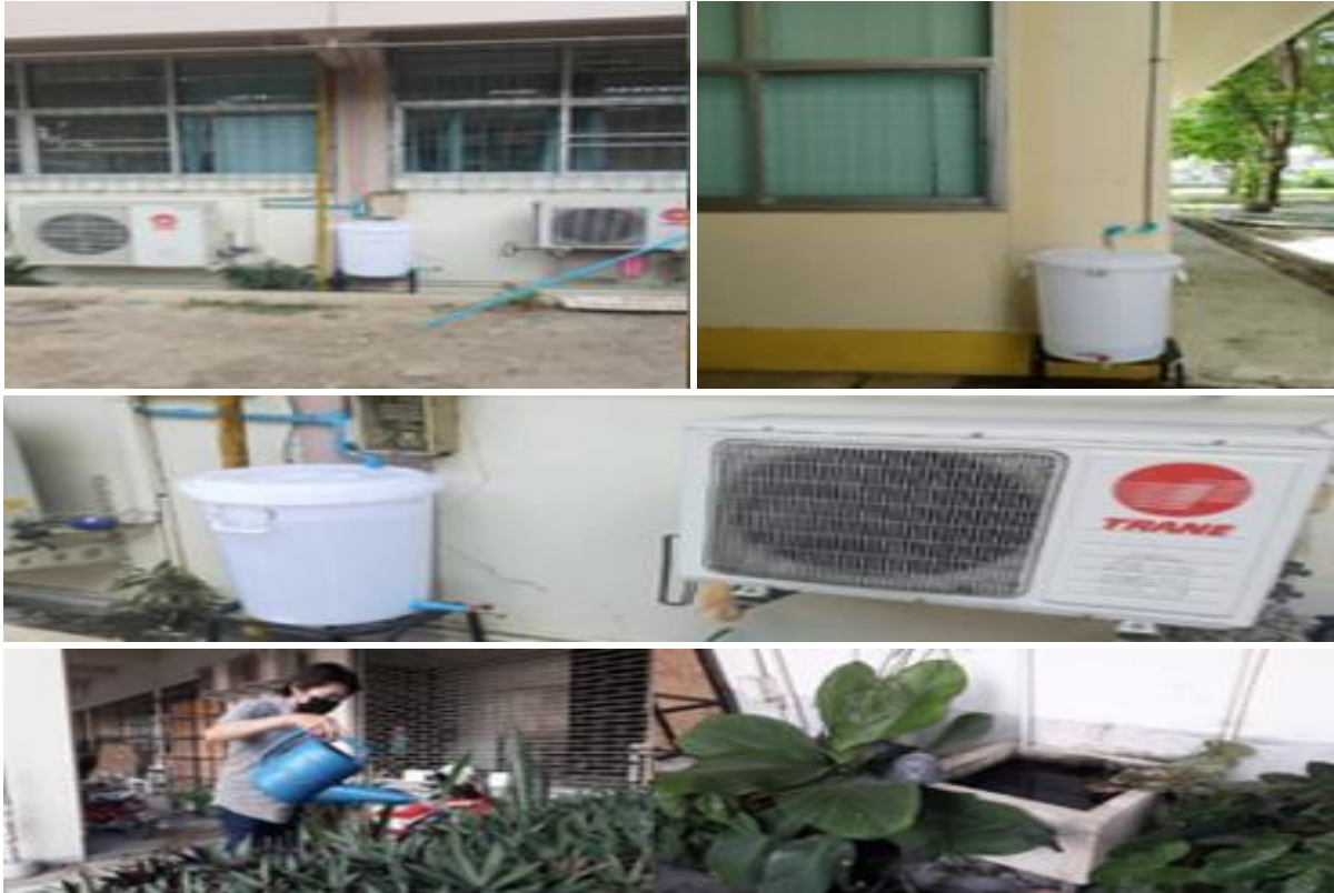
Water collection from air conditioning systems
