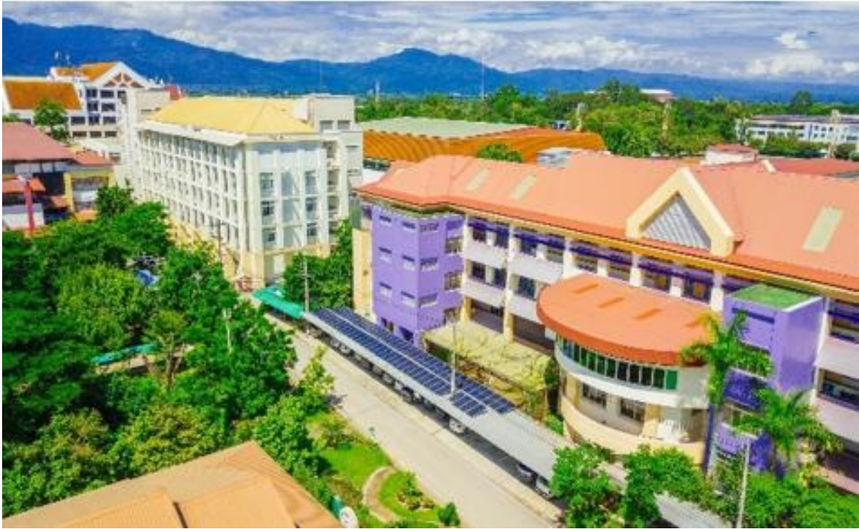
Solar panels with 20-kW installed capacity at a parking lot.
