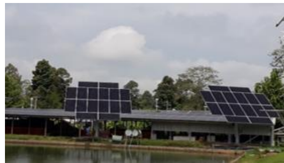
A solar tracking station with a capacity of 20 kW has been erected
