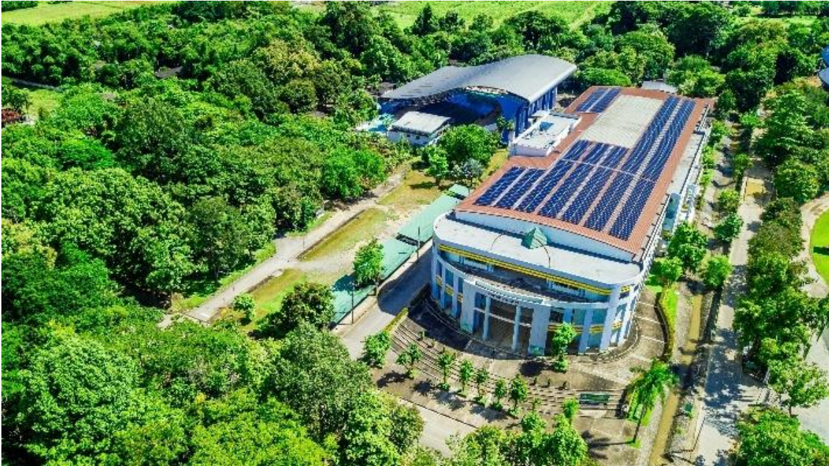
Solar panels with 300-kW installed capacity on the roof
