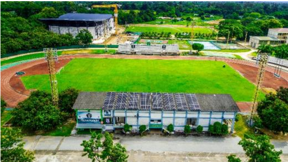
Solar panels with 40-kW installed capacity at the stand
