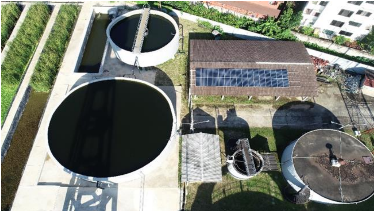
Solar panels with 10 -kW installed capacity on the roof
