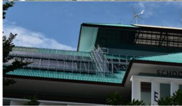
Solar rooftop with a 300-kW capacity on a renewable energy classroom building
