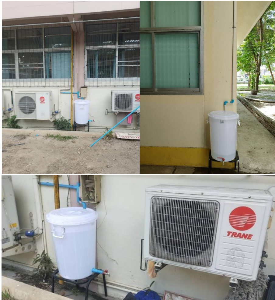
Water collection from air conditioning systems at Office of the President building
