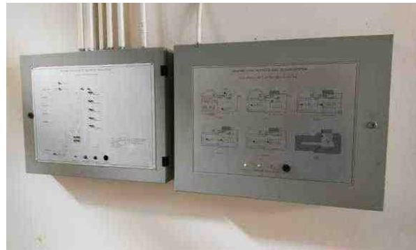
Graphic Annunciator informs the location of the incident in the building.
