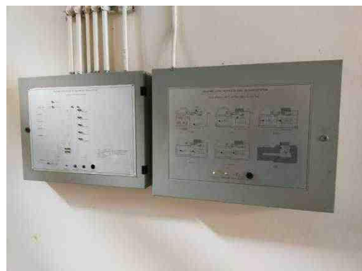
The graphic Annunciator informs the location of the incident in the building.
