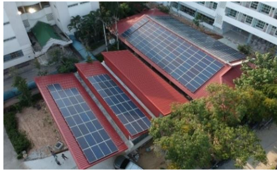
Solar rooftop with 80-kW installed capacity
