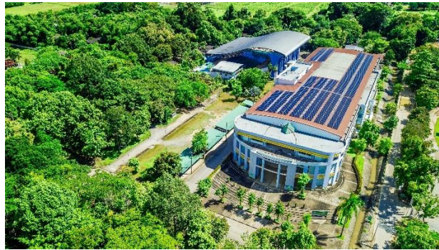
Solar panels with 300-kW installed capacity on the roof
