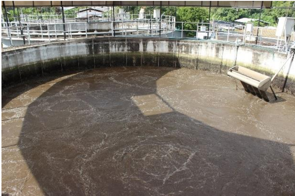
SBR reactor tank (Full capacity 2400 M3. / day)
