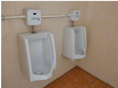
waterless urinals and automatic urinals
