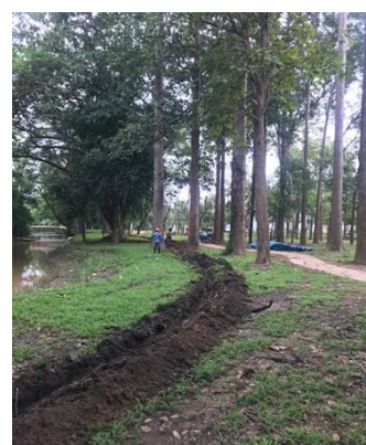
Laying Treated wastewater pipes into the garden
