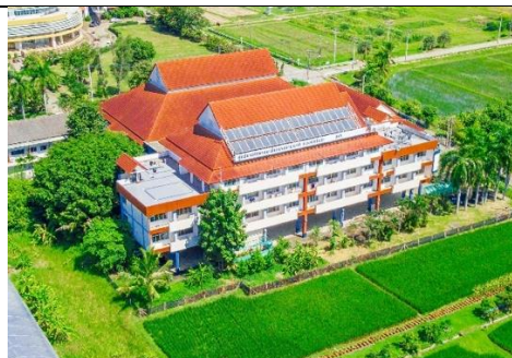
The International Education and Training Center's roof is covered with solar collectors and an installed capacity of 84 m 2 tanks.
