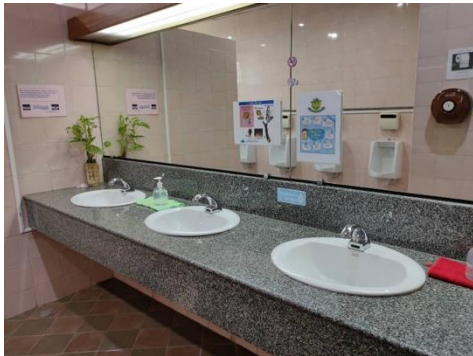
low flow taps and automatic taps
