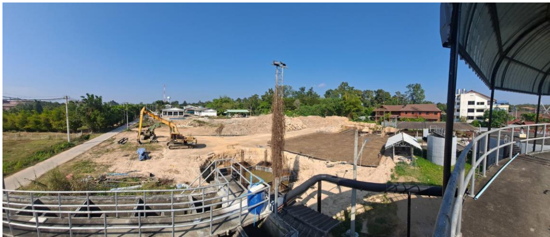
Construction of sewage treatment and wetland system (in progress)
