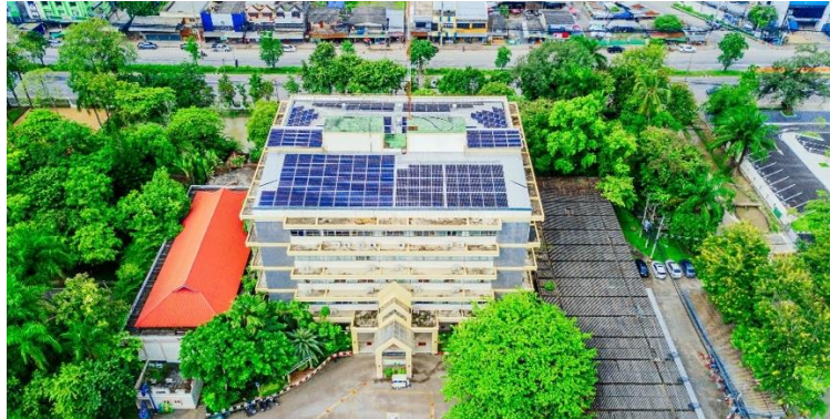
Solar rooftop with a 110-kW installed capacity
