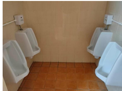
waterless urinals and automatic urinals
