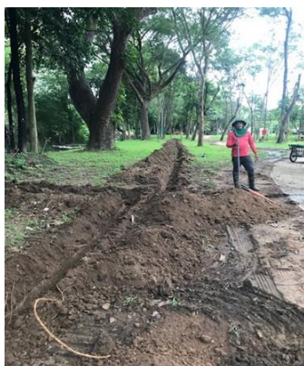
Laying Treated wastewater pipes into the garden
