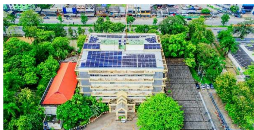
Solar rooftop with a 110-kW installed capacity
