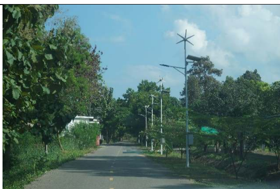
For street lighting, 35 units of hybrid system of solar and wind turbines are used, School of Renewable Energy
