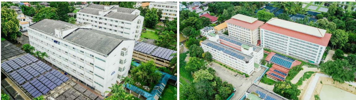
Solar collectors' panels with 1331 m 2 installed capacity and tanks on Students' Dorm All Student Dormitories
