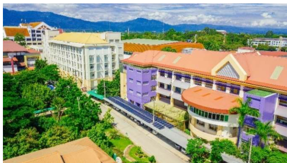
Solar panels with 20-kW installed capacity at a parking lot, Faculty of Economics
