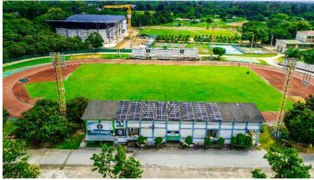
Solar panels with 40-kW installed capacity at the stand, Inthanin Stadium's Stand
