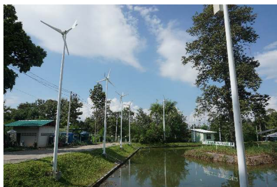
On the school of renewable energy, wind turbines with a total capacity of 16.5 kW generate electricity.
