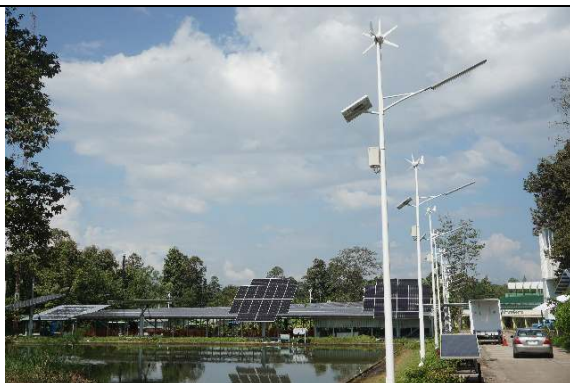
For street lighting, 35 units of hybrid system of solar and wind turbines are used. (cont.)
