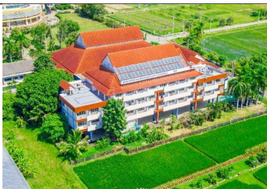
Solar collectors' panels with 84 m 2 installed capacity and tanks on Students' Dorm, International Education and Training Center
