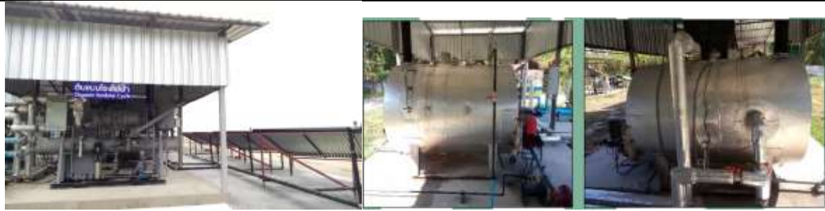
Scope 1: stationary combustion to burning of fuels to produce electricity by Organic Rankine cycle (ORC) technology using solid wastes at MJU
