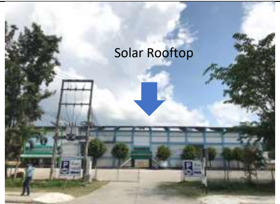
Solar rooftop station 2 capacity electricity of 40 kW
