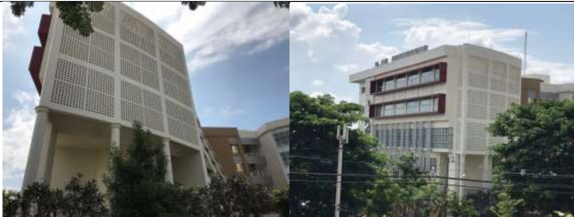
Full natural daylight in building
