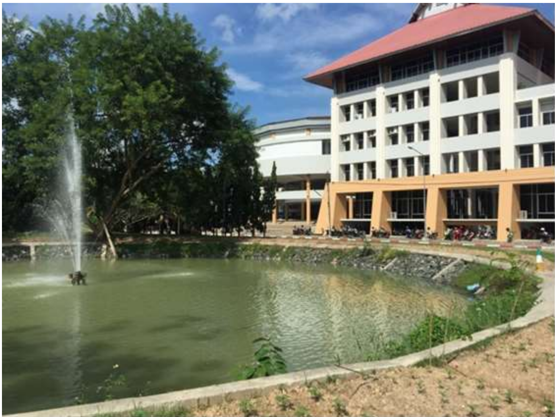
Treated wastewater released to the pond
