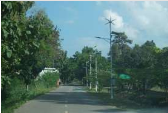
Solar and wind turbine hybrid system for street lighting about 35 units
