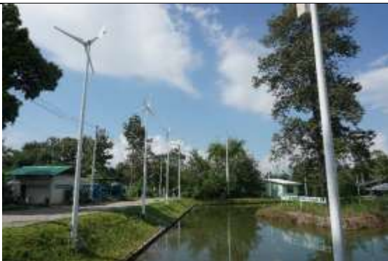
Wind turbine power generation, total capacity of 7.5 kW at MJU
