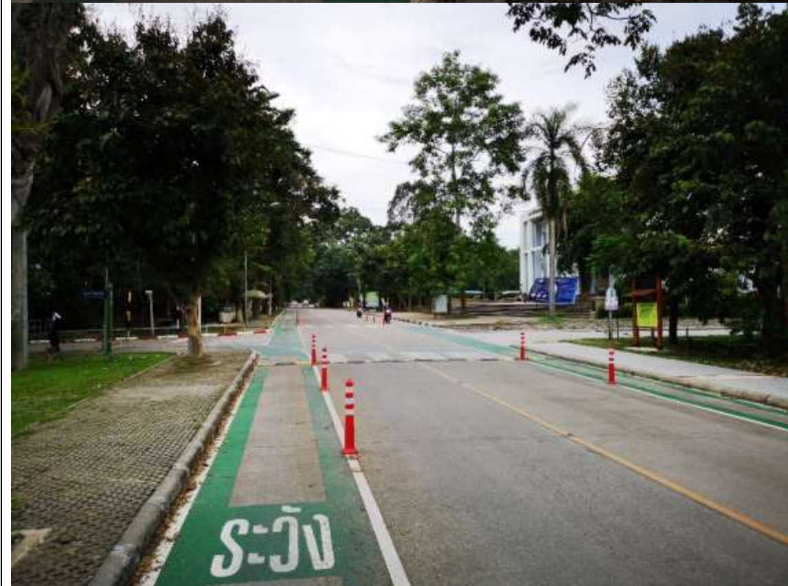
The pedestrian path on the main road of the campus (Intanin Rd.) has separated from road, leveling up platform, enough space, channelized control at intersection, and surrounding with nature
