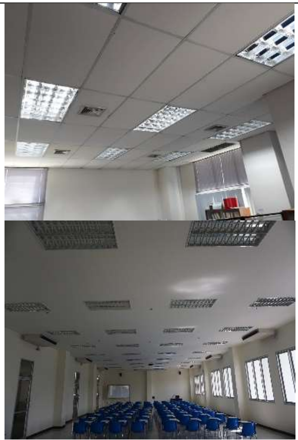
Replacing LED + T5 lighting fluorescents about 43,803 units in MJU
