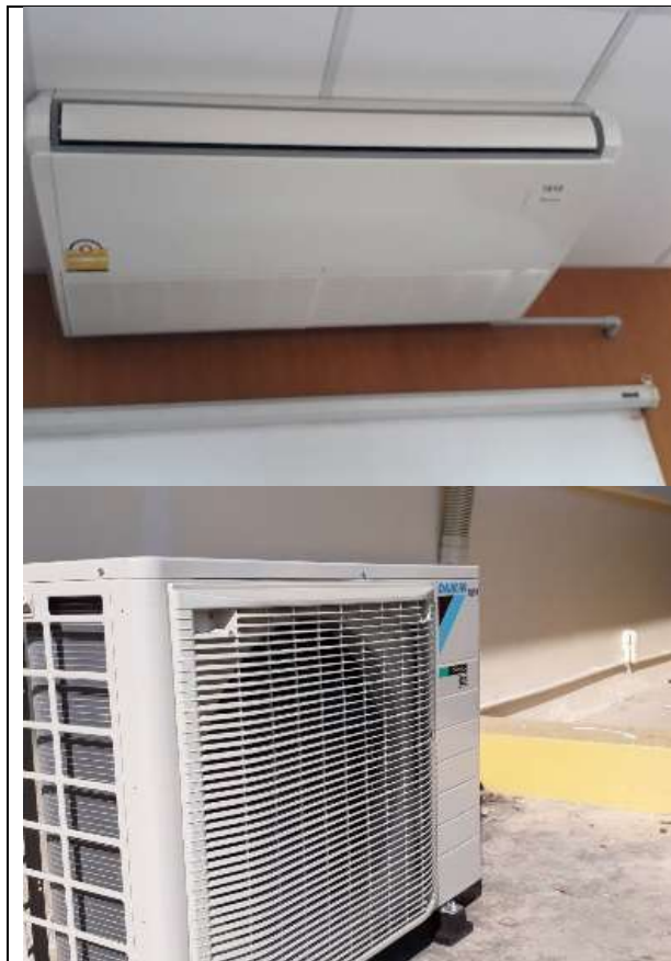
Replacing air-conditioning high efficiency (Label No.5) about 454 units MJU
