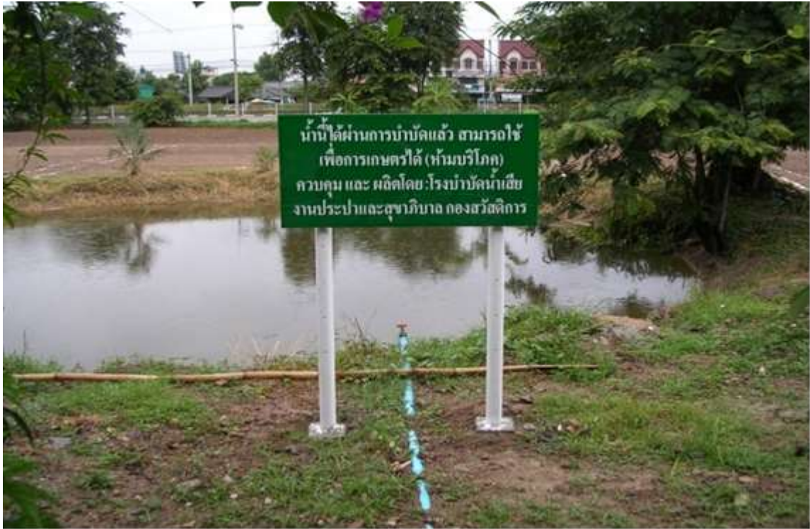
Treated wastewater released to the pond
