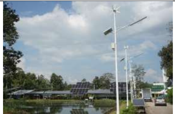
Solar and wind turbine hybrid system for street lighting about 35 units
