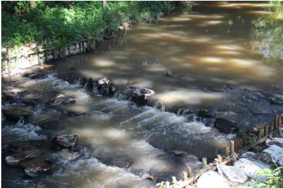
Weir in the natural canal
