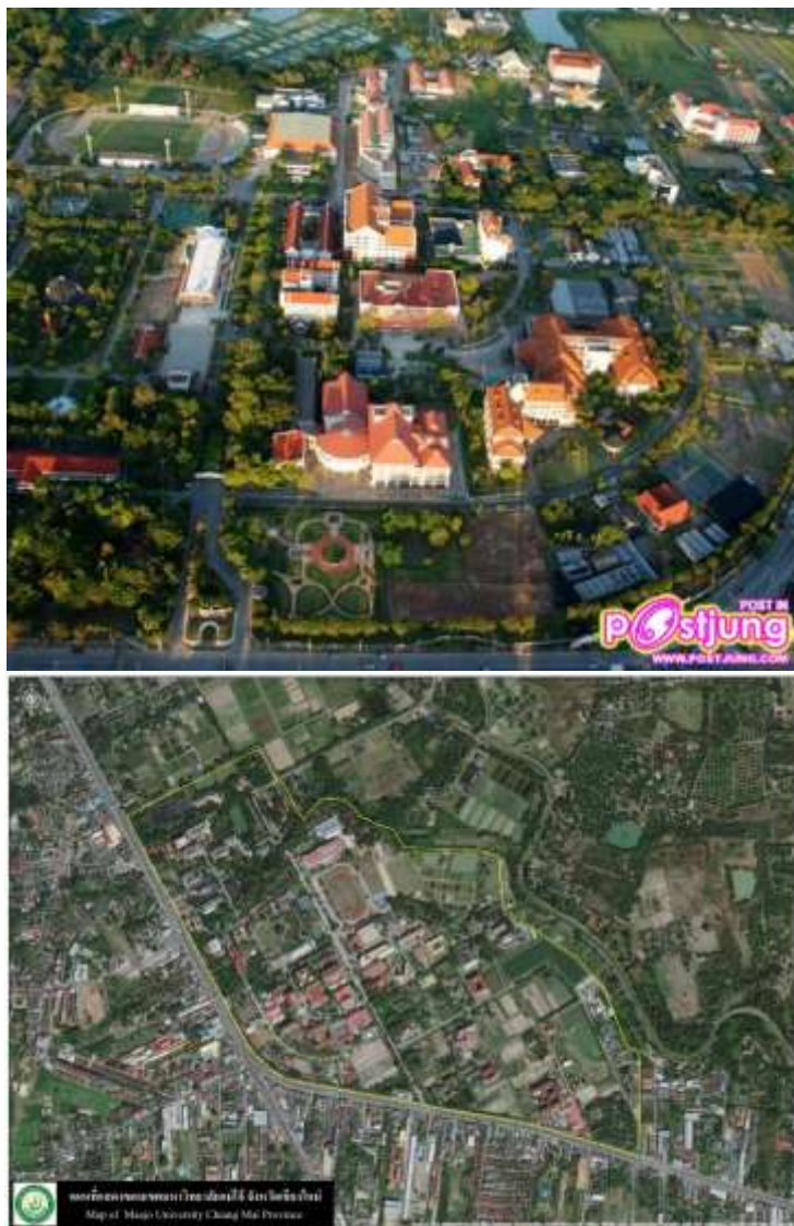
MJU Chiangmai campus (Main Campus) 1,280,000 m 2 building, farm, garden and forest
