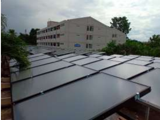
Solar water heating station 1, area installed of 1,313 m 2 at Student Dorm Building
