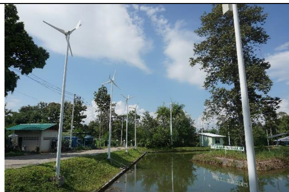
Wind turbine power generation, total capacity of 16.5 kW at MJU
