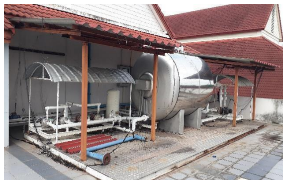
Energy storage of solar water heating on International Education and Training Center
