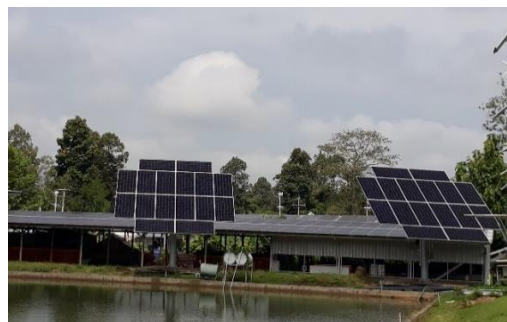
Solar tracking station installed with capacity of 30 kW
