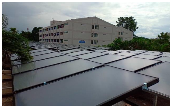
Solar water heating station 1, area installed of 1,313 m 2 at Student Dorm Building
