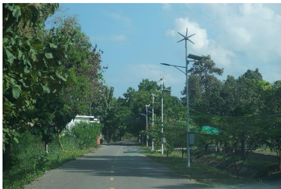
Solar and wind turbine hybrid system for street lighting ( 35 units)
