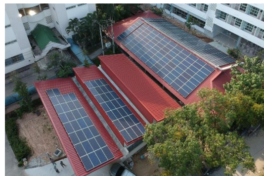
Solar rooftop installed capacity of 80 kW
