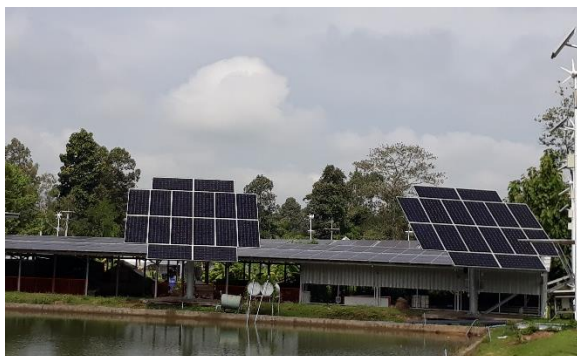
Solar tracking installed capacity of 30 kW
