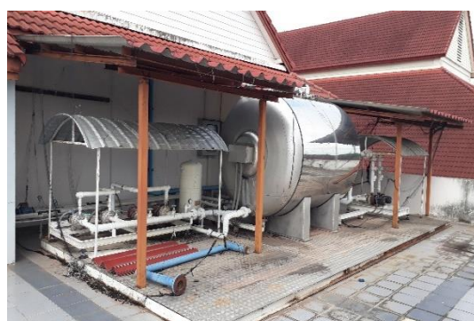
Energy storage of solar water heating on building
