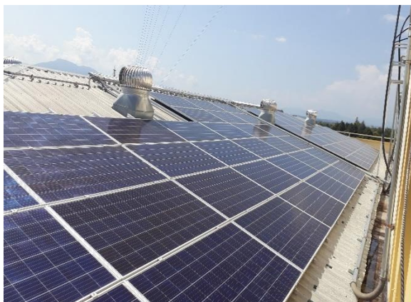
Solar rooftop with the installed capacity of 20 kW
