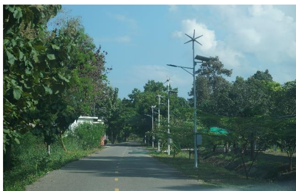
Solar and wind turbine hybrid system for street lighting ( 35 units)
