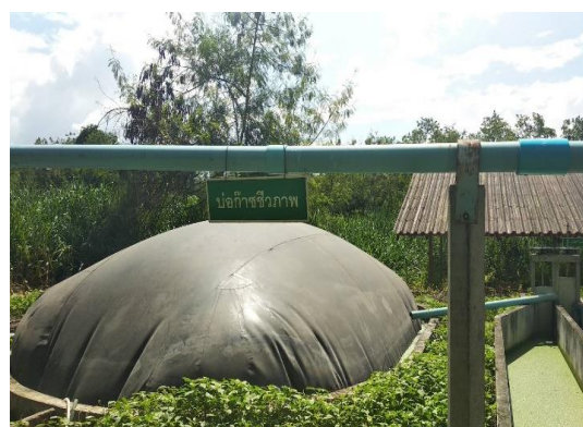
Biogas production system with the capacity of 300 m 3 for electricity generation
