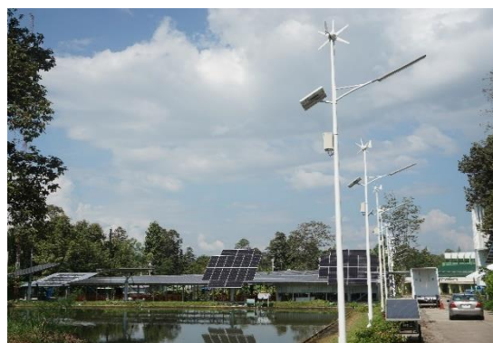
Solar and wind turbine hybrid system for street lighting (35 units)
