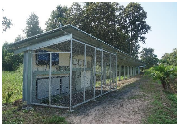
Solar rooftop at parking installed capacity of 40 kW
