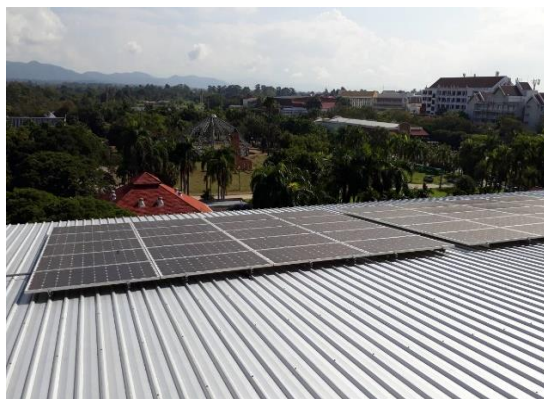
Solar rooftop the installed capacity of 90 kW
