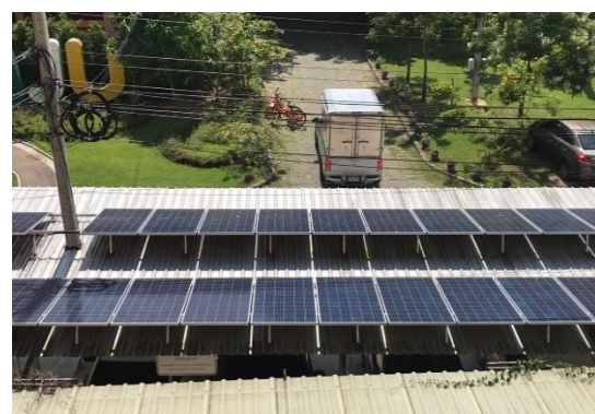
Solar rooftop at parking installed capacity of 20 kW
