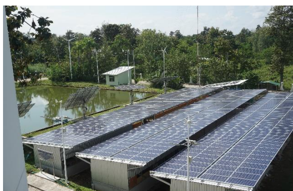
Solar rooftop at Renewable Energy Laboratory Building installed capacity of 300 kW
