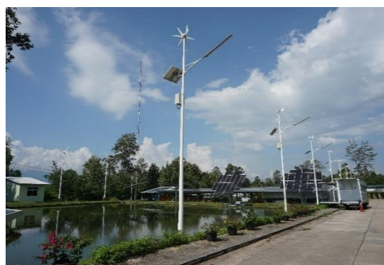
Wind turbine power generation, total capacity of 7.5 kW at MJU
