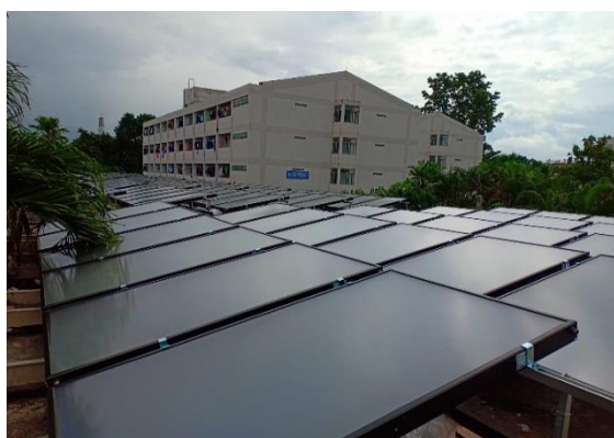
Solar water heating station 1, area installed of 1,313 m 2 at Student Dorm Building
