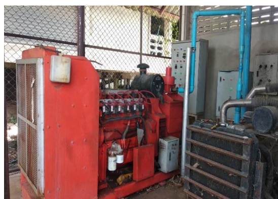
Biogas engine for power generation
